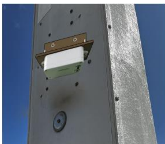
Figure 1. Install the device upside down.
