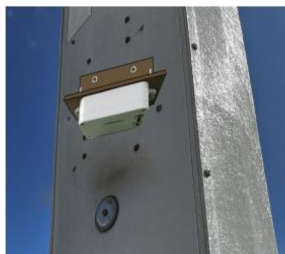
Fig 2. Install with LED and function key faced downwards
